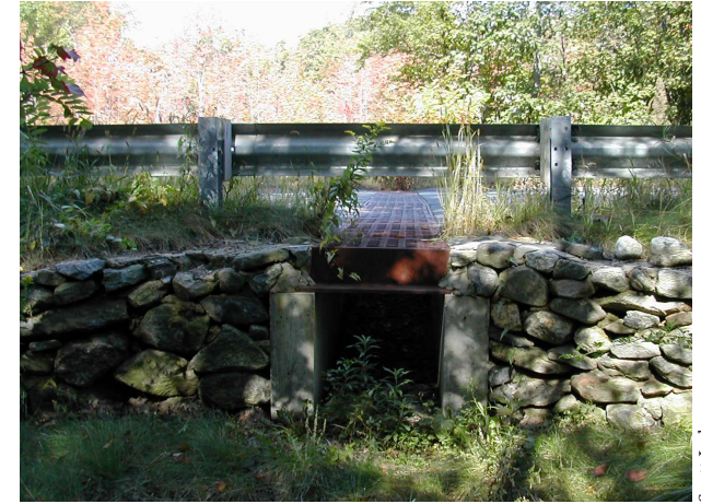
Road passage structures allow organisms such as turtles and salamanders to access habitat without crossing roads.
