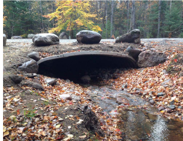
Wide culverts allow aquatic organisms to more readily pass beneath roads.
